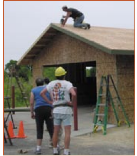
2009 Park Hero, Duane Deutmeyer, stains fascia board on the firewood building.
